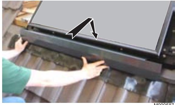
8. Tighten the screws to hold the housing in place. Do not block in order to adjust the position of the housing at the end of assembly.
